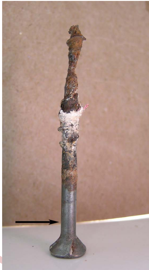
Figure 3. Cabinet screw as-received. Note the base still retains the zinc coating while most of the material was corroded away due to exposure to water and a more noble copper.
